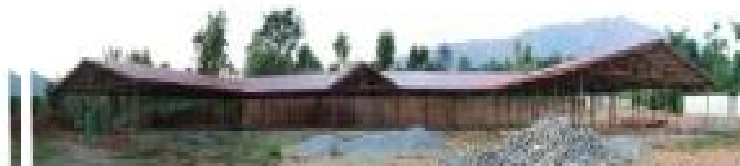
November 2017: the new 50-bed hospital being built Planned opening - Nov. 2018 (Funding dependent)
